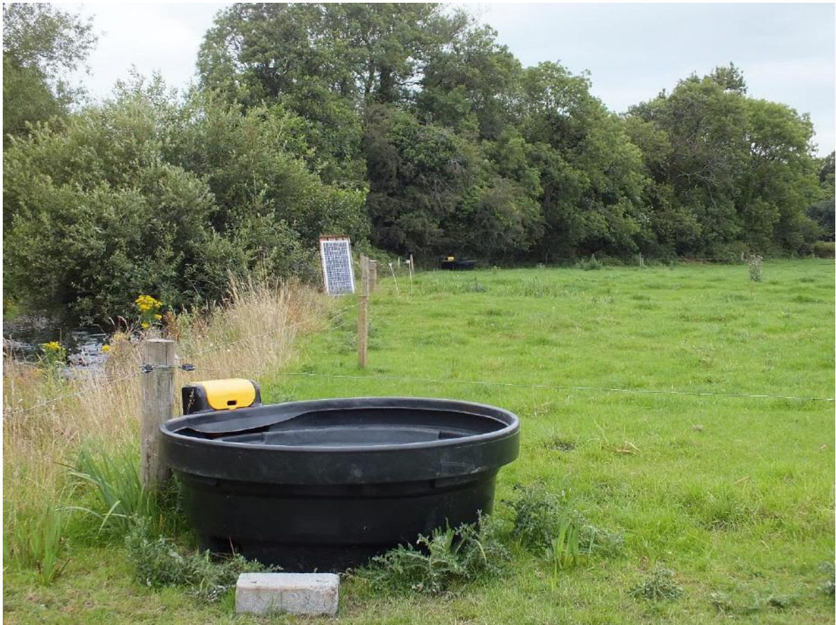
Figure 5 Solar panel in the middle-ground powers the machine that pumps water from the river to either of the two drinking troughs (foreground and background) – demonstration farm (dairy)
